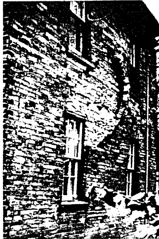
FIG. 26. Damage to opposite side of the two-story residential unreinforced masonry dwelling of Fig. 25 (Berkey 1945).
