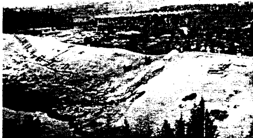
FIG. 19. Slide of railroad embankment near Parent, Quebec, some 350 km from the epicentre (photo by Canadian National Railways, Geological Survey of Canada archives).
