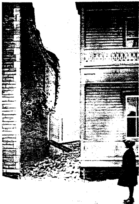
FIG. 12. Out-of-plane failure of unreinforced masonry wall in Shawinigan (Laroche 1982).
