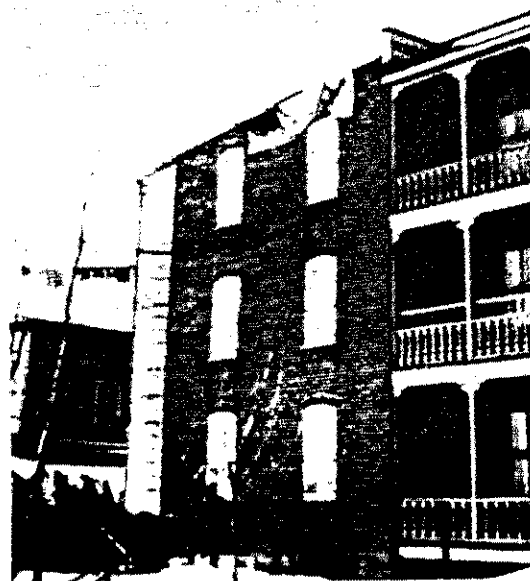
FIG. 11. Out-of-plane failure of unreinforced masonry wall in Shawinigan, approximately 250 km from the epicentre (Hodgson 1950).
