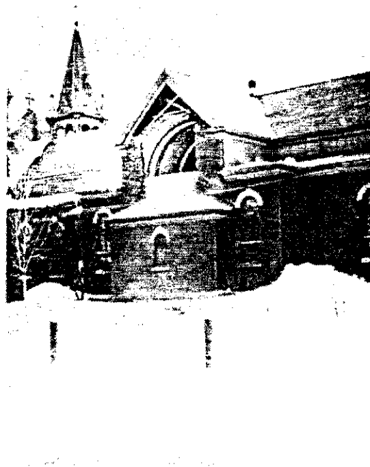
FIG. 13. Out-of-plane failure of unreinforced masonry transept wall of St. Marc Church in Shawinigan (Geological Survey of Canada archives).
